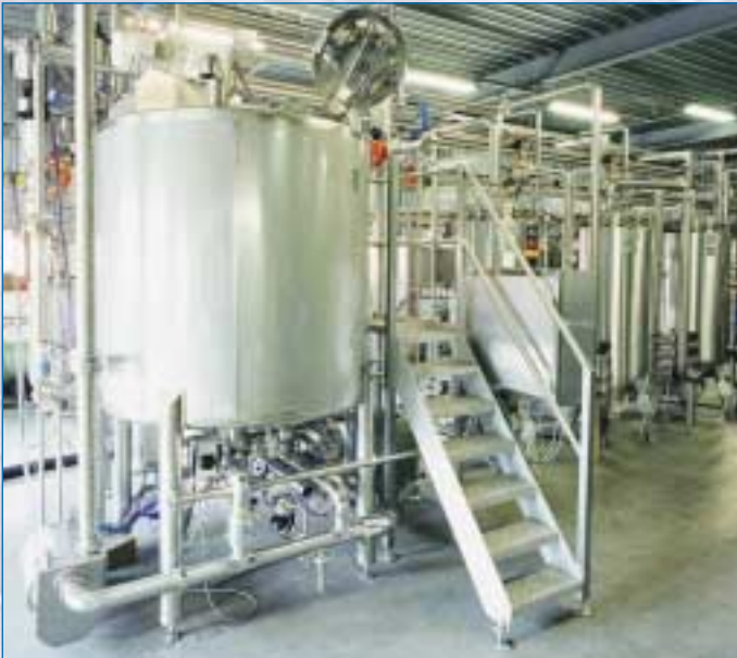
Installation of a sauce line
