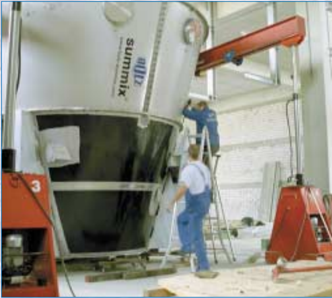
Installation of a conical mixer
